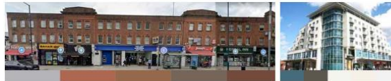
The Quadrant (81-167 Station Road) Inter-war shopping parade, 1928 Three storeys Red brick Commercial frontage ground floor Built for Cohen and Cross (company of the developer George Cross)
