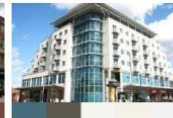
Centurion House Site of demolished Ritz Cinema Seven storeys Whitefaced render, large glass panels Mixed use - residential with commercial on ground floor
